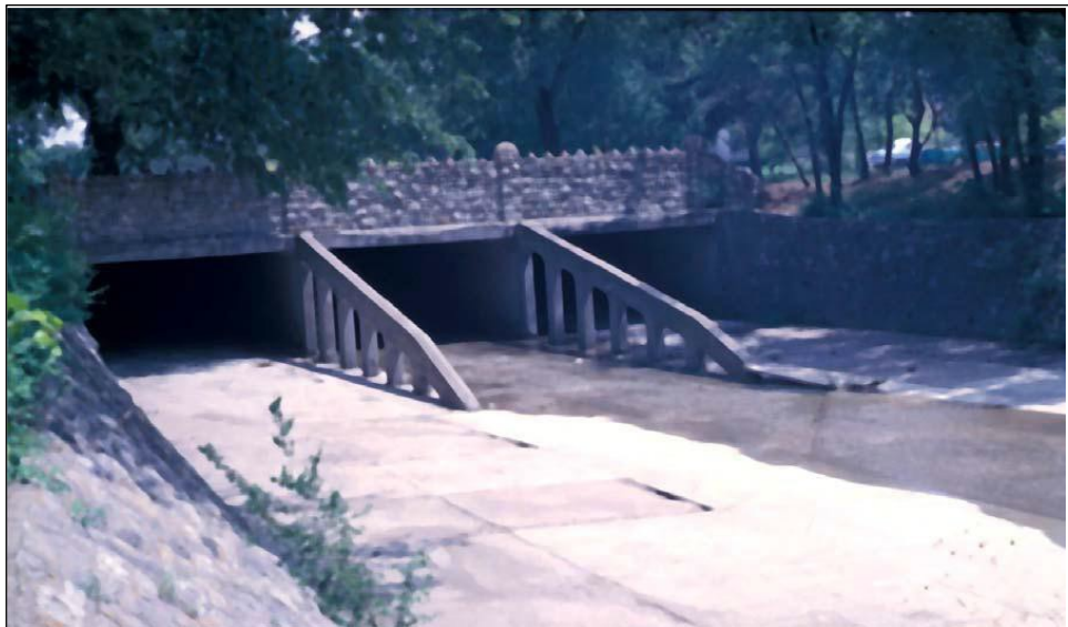
Figure 1. Debris fins upstream of bridge piers (NCHRP 653)
