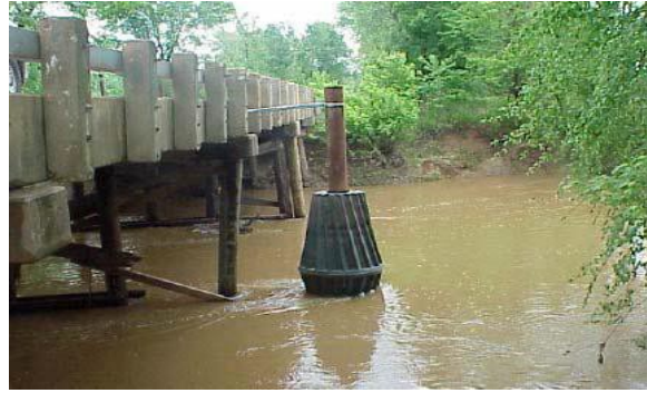
Figure 2. Debris Sweeper Installed Using Pier Attachment (Bradley et al. 2005)
