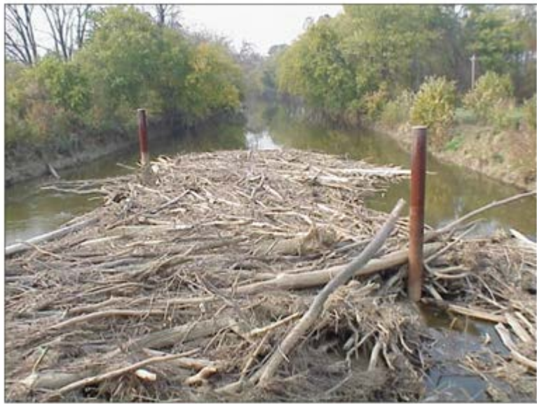
Figure 3b. Debris accumulation at the column debris deflectors (Lyn et al 2003)
