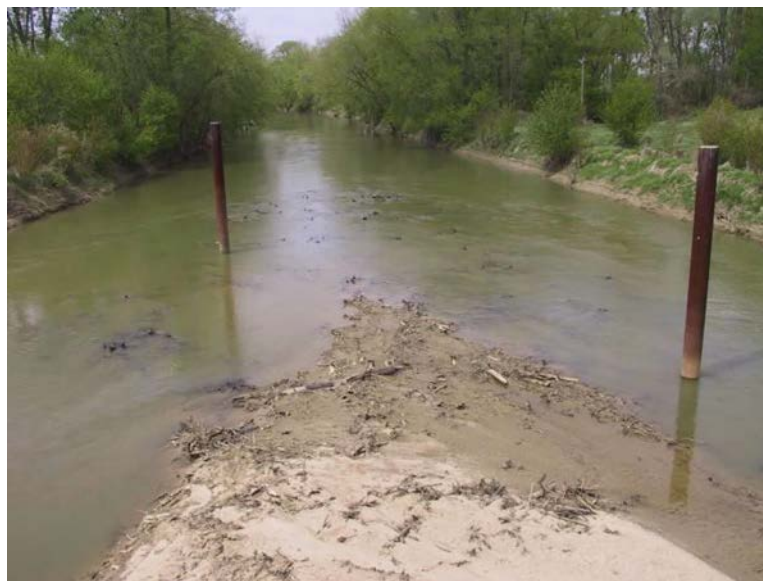
Figure 3a. Cylindrical Pile debris deflectors installed in an Indiana River (Lyn et al 2005)
