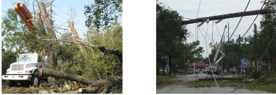
Figure 1. Falling Down Trees Caused Damages to Electrical Poles (Center-Point Energy)
